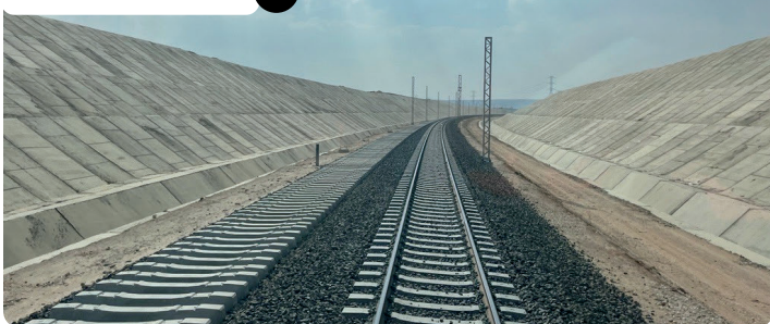
LGV "green line" 2023-en cours 🇪🇬
